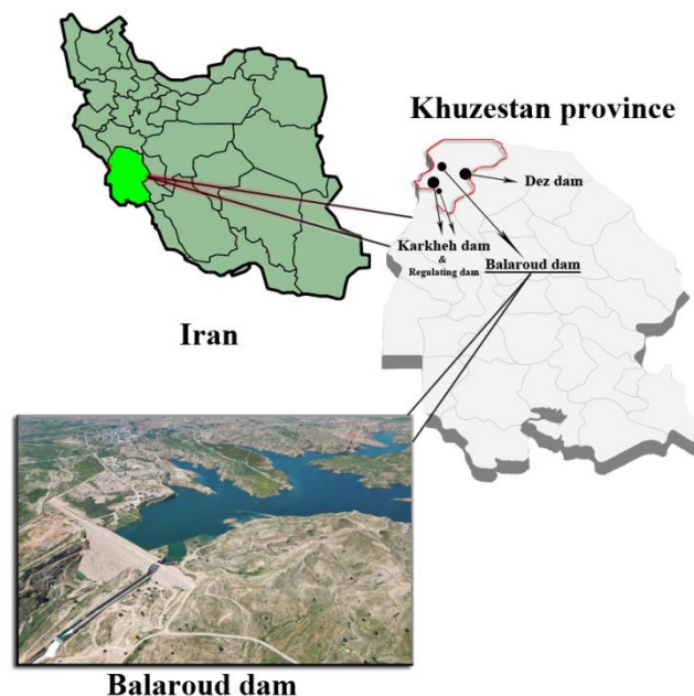
Fig. 1. Location of the Balaroud reservoir dam.
