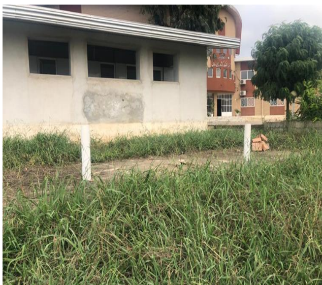
Fig. 2. Septic tank buried in land.
