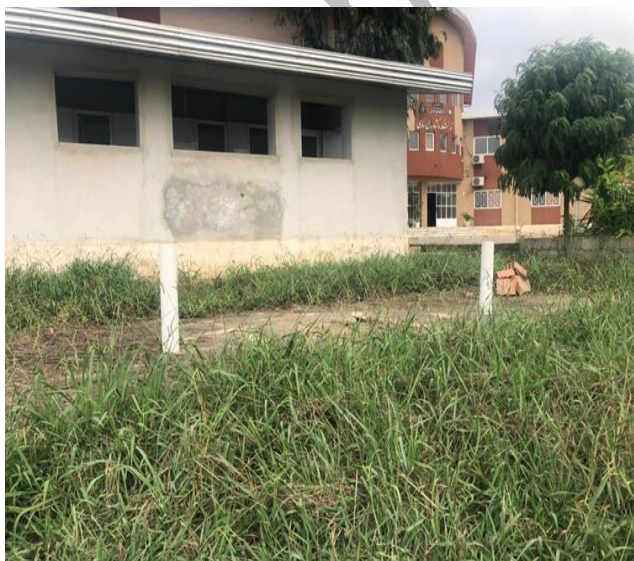
Fig. 2. Septic tank buried in land.
