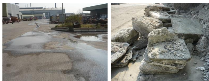
Fig. 1. First flush stormwater collecting on hard-stand areas at the smelter site (left) and solid lead waste on the ground at the smelter site (right).
