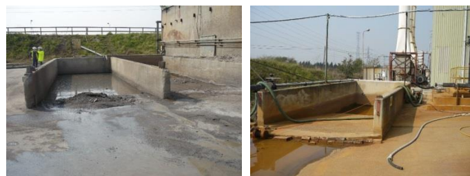
Fig. 2. Stormwater collection and settling bays, for lagoon #1 (left) and for lagoon #2 (right).
